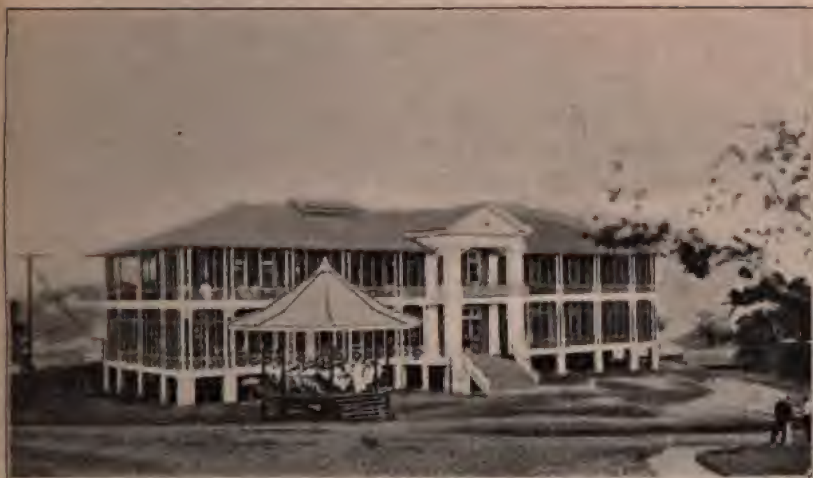
FIG. 9.— Club-house at Culebra, Panama, showing construction for thorough screening against mosquitoes.
